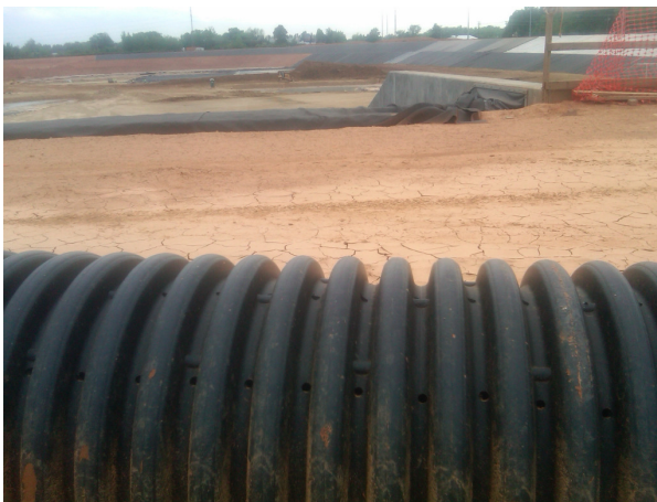
Corrugated HDPE pipe with a Class II perforation pattern enables water to enter the long-life system and be conveyed to a central collection point.
